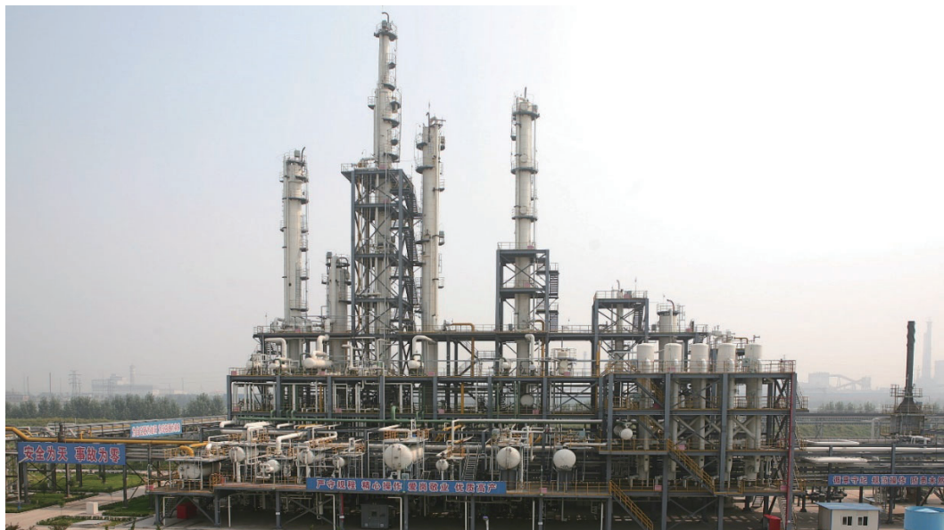
Crude benzene hydro-refining facility at our Xingtai Production Base
