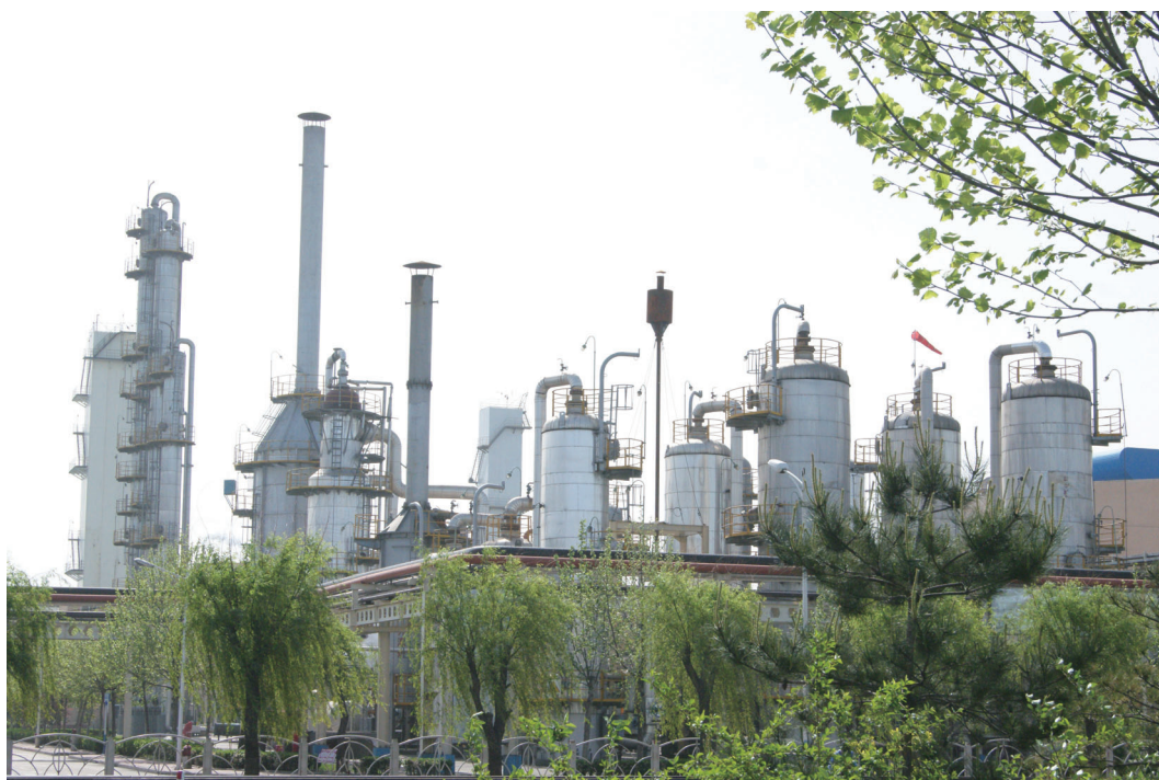
Methanol production facilities at our Dingzhou Production Base
