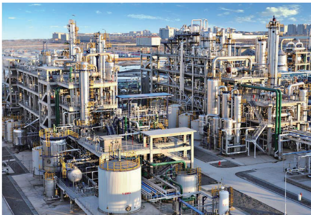
Caprolactam production facilities at our Cangzhou Production Base
