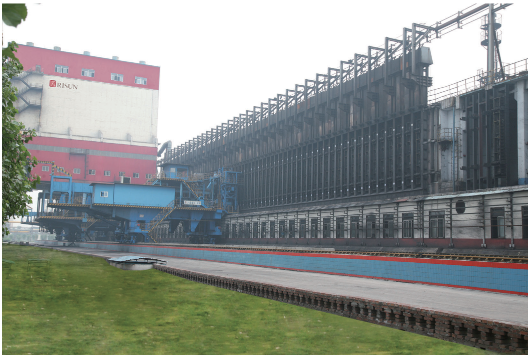
Coke facilities at our Dingzhou Production Base
